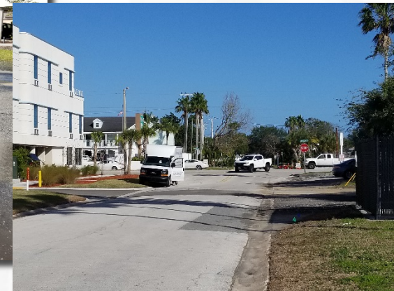
Dry roadway after one-way tidal valve installation
