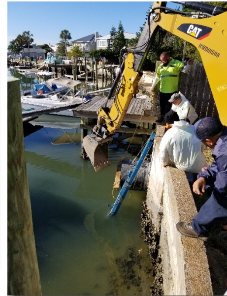
City installation of one-way tidal valve in FDOT outfall
