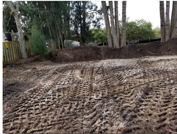
Coquina Park grading work
